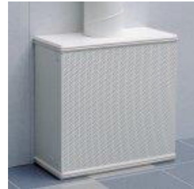
Displacement ventilation in auditorium
