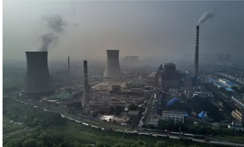
▲ A state-owned coal-fired power plant in Huainan, Anhui province, China. Photograph: Kevin Frayer/Getty Images
